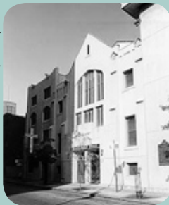
The Second Baptist Church, which still stands at 441 Monroe Street in Detroit.
